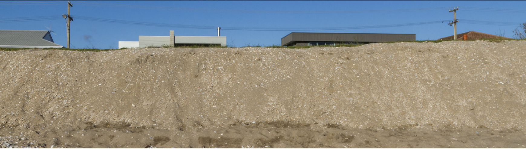
Dune erosion at Buffalo Beach, Whitianga
