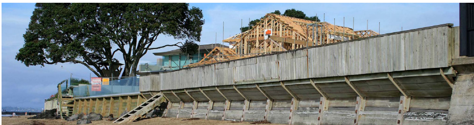
Protective works and redevelopment on the shoreline at Milford, Auckland
