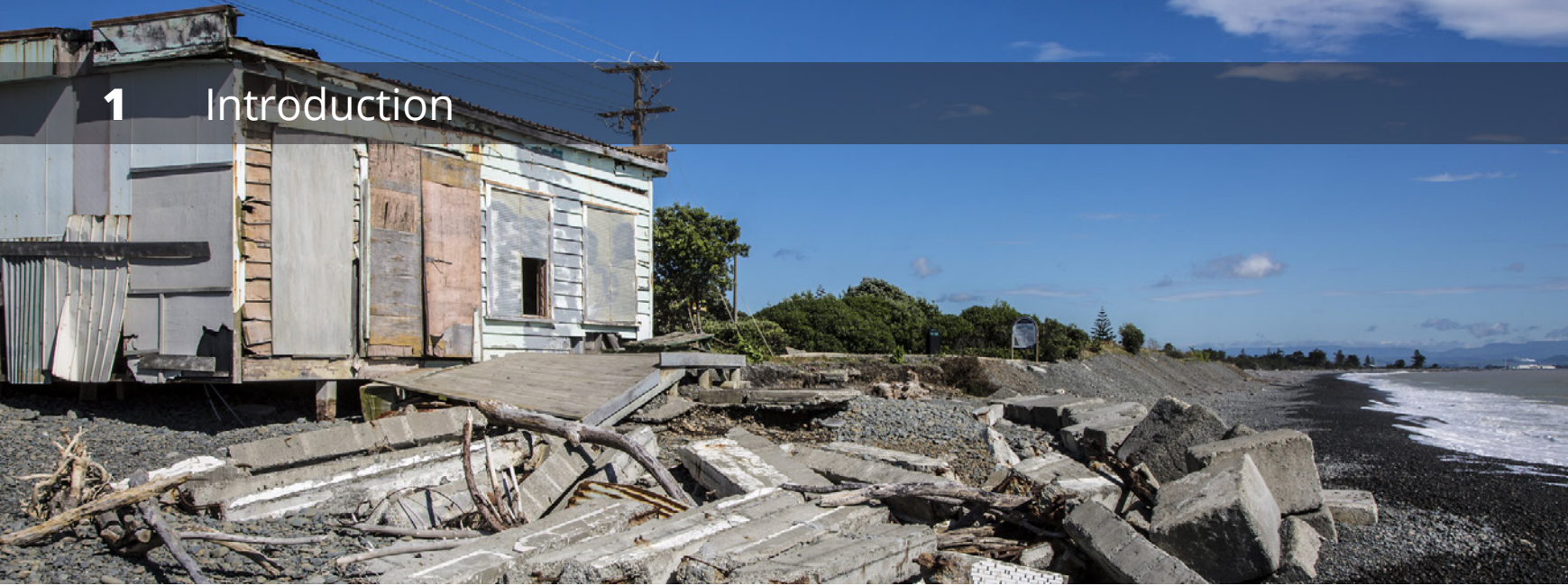
Coastal erosion damaging a house at Haumoana
