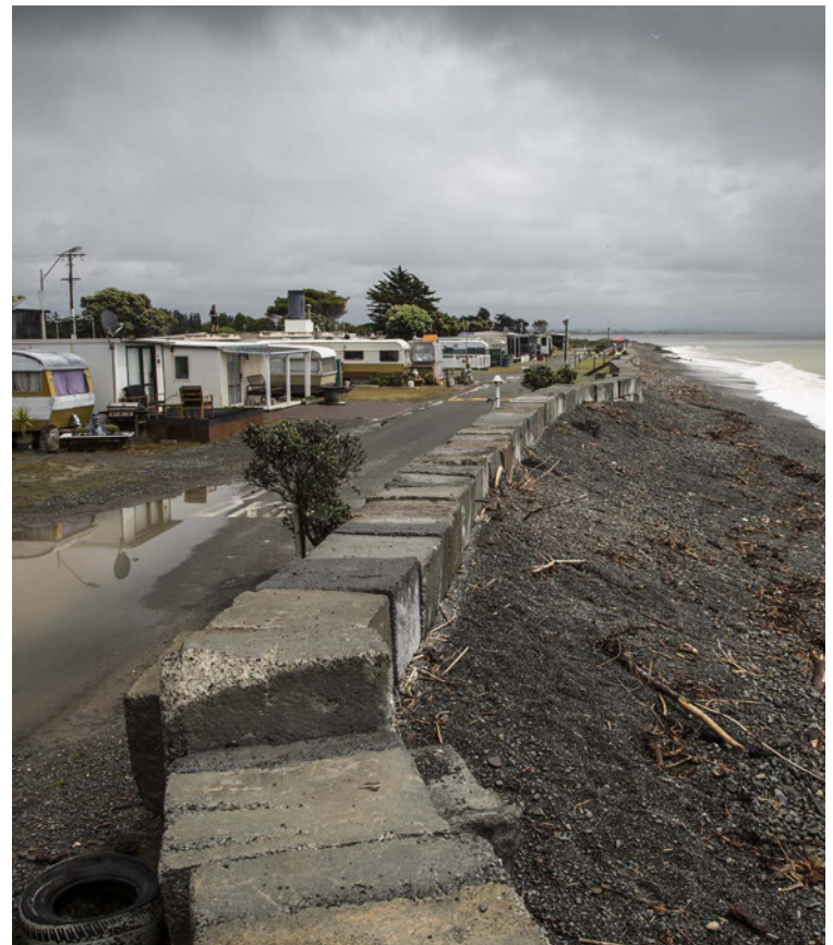
Coastal erosion impacting the Clifton Motor Camp
